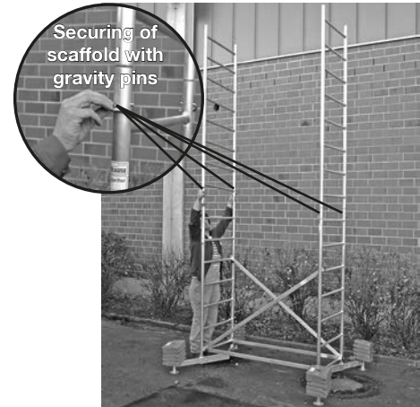
Basic frame with first and second extension
