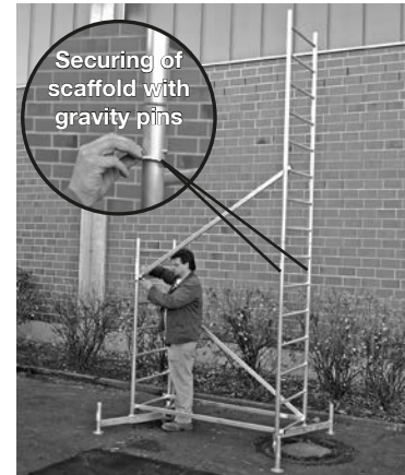
Basic scaffold with first extension
