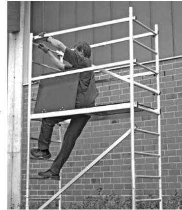
Basic scaffold with first extension
