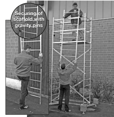
Basic scaffold with first and second extension
